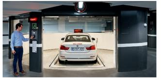
The car transfer section is equipped with a monitor, which displays whether the vehicle has been correctly positioned. The vehicle height, width and length are monitored to make sure that the vehicle dimensions are compliant with the system configuration parameters. As soon as all the data has been verified, the driver is prompted via the monitor and can climb out of the vehicle.
