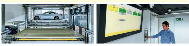
Due to the complex building circumstances, two of the systems have been additionally equipped with a lateral vertical lift which can also be reached effortlessly by the car transfer areas for car parking and retrieval operations. Car parking operations are thus performed dynamically, whereby the empty stacking position found closest to the car transfer area is occupied first.
